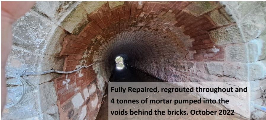
New Brick to fill voids and to replace damaged, metal inserts to reinforce Arches. October 2022
