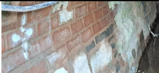
New Brick to fill voids and to replace damaged, metal inserts to reinforce Arches. October 2022
