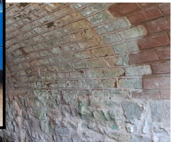
New Brick to fill voids and to replace damaged, metal inserts to reinforce Arches. October 2022
